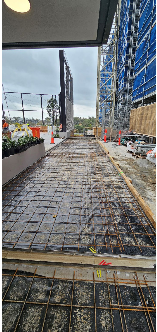
Forming for topping slab, School level 1
