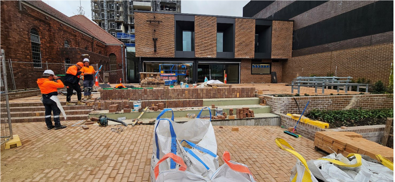
Paving of bleachers – Parish Forecourt
