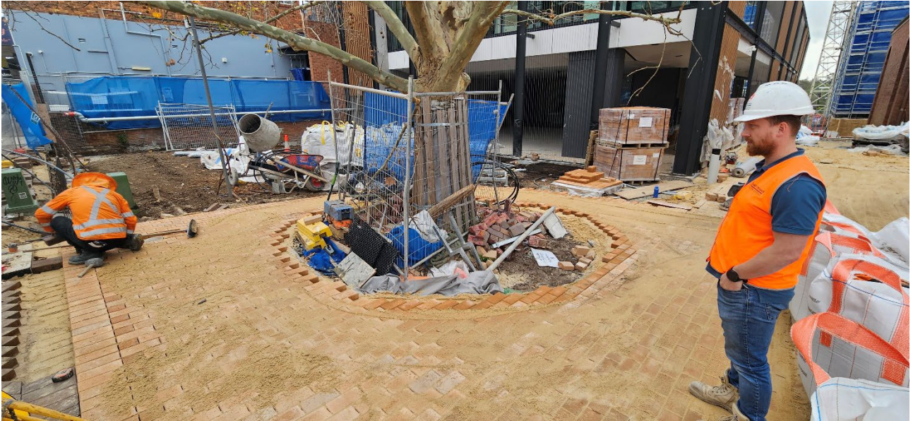
Paver install – School, Oxford St frontage
