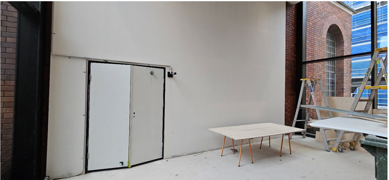
Temporary fire door hold-open installation - Link Bridge Parish Hall/Church
