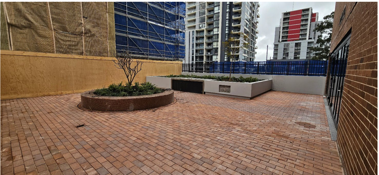
Paver install and soft landscaping - Parish Courtyard, Level 1
