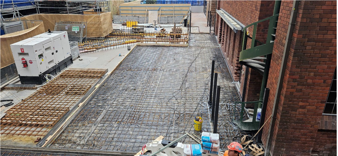
Forming for topping slab – OSHC, Level 1
