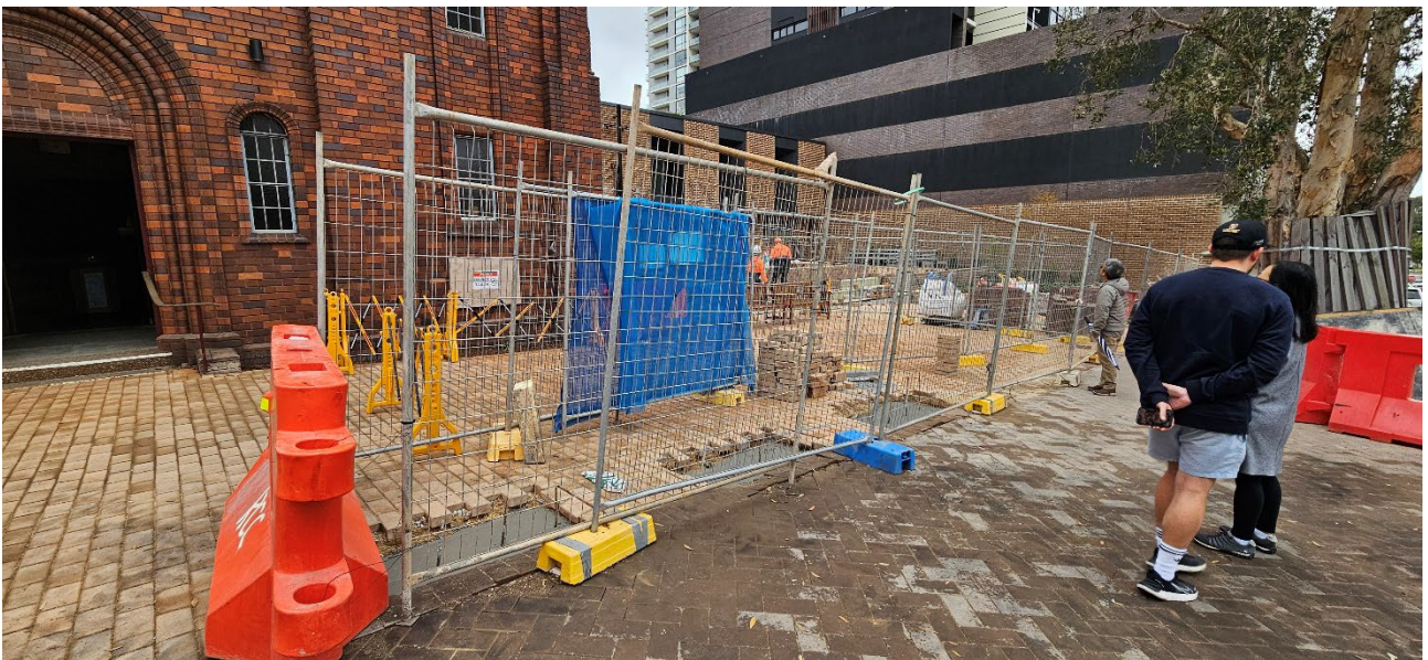
Crash barrier construction – Church, Oxford St frontage
